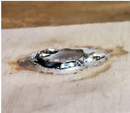
Spot weld on bottom plate
